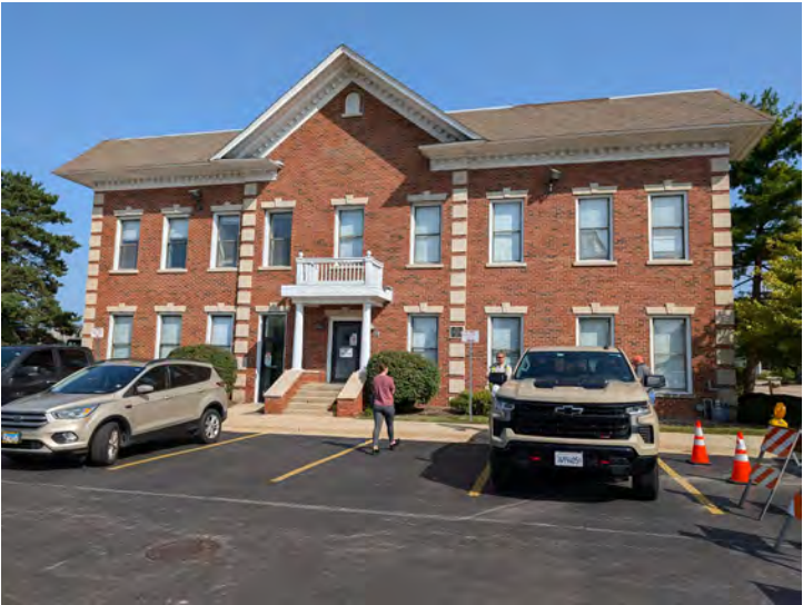
VIEW OF SOUTH FACADE
