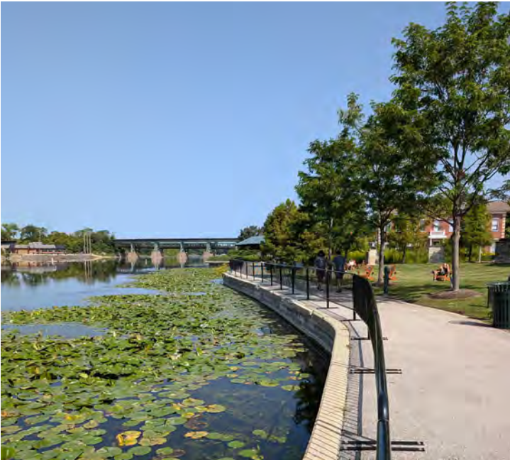
2 VIEW OF RIVER EDGE WALL
