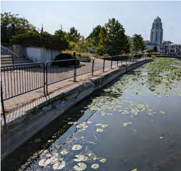
1 VIEW OF RIVER EDGE WALL
