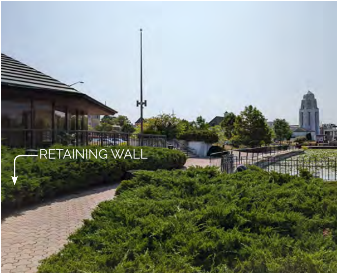
3 VIEW OF RETAINING WALL (behind planting)
