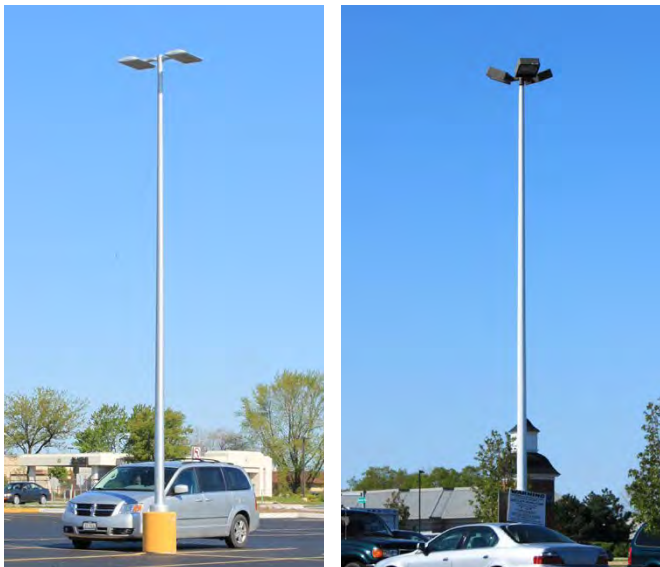
Images above depict two types of parking lot lighting. The image on right (discouraged) is flood lighting, where fixtures flood areas, requiring fewer fixtures but contributing to light pollution. The image on the left (encouraged) directs light downward minimizing spillover lighting.
