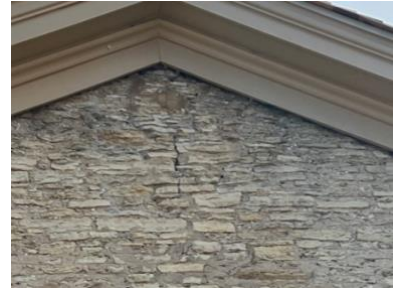
Figure 17. Close-up highlights cracked mortar joints.
