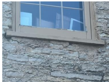
Figure 14. Cracking mortar detected, requiring injection to fill voids – 2 floor
