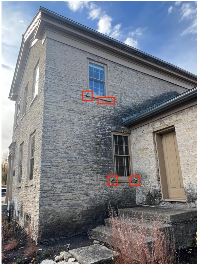
Figure 12. North elevation showing areas with open voids.
