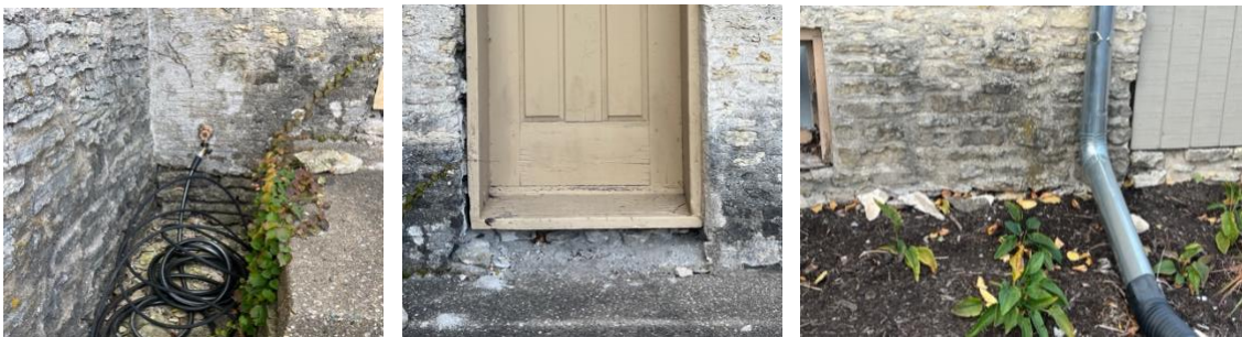
Figure 9-11. Cracking mortar detected, voids under door sill and open joints at the foundation
