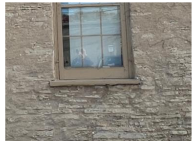
Figure 18. Open voids in the windowsill masonry.
