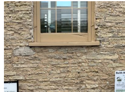
Figure 2. Close-up showing open voids in the windowsill on the East elevation.
