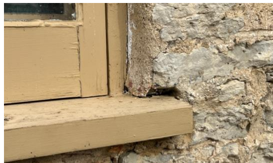
Figure 7. Close-up showing open voids in the windowsill at the South elevation.
