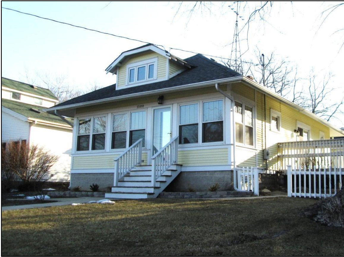
19. 1508 Riverside Avenue Sears "Starlight"
