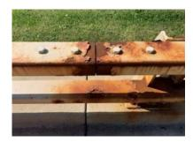
No structural damage was observed in the railings. A majority of the reflectors attached to the top rail are broken, bent, and/or corroded. Rust staining is typically observed along the concrete curb line.
