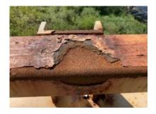
The ends of the railing tubes exhibit corrosion and section loss at splices, while the bolts are in good condition.
