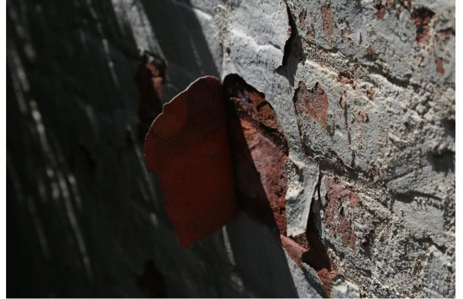
The face of the brick is failing in places and the paint is peeling because of it. It needs the attention of a masonry expert to preserve the brick and provide a decent surface to paint. These are just a couple small spots. There is a larger spot that was too high to be easily photographed.
