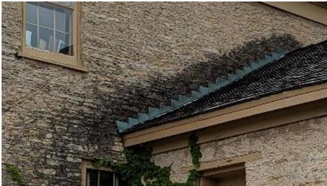
*Damage to limestone on north façade*
