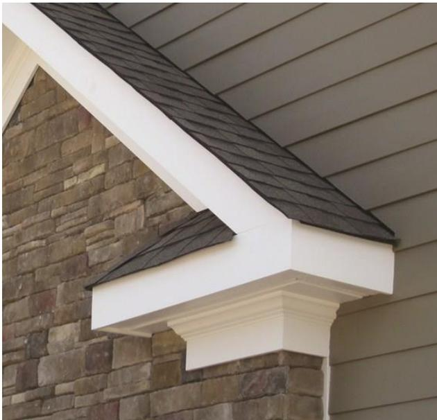
*Example of soffit, fascia, and crown molding in Poly-ash*
