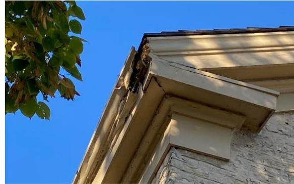
*Damage to south crown molding, fascia, and soffit*
