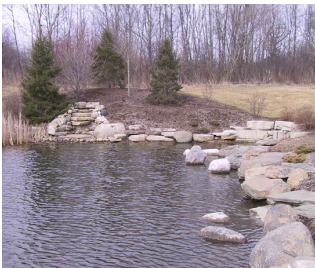
Wet Stormwater Detention
