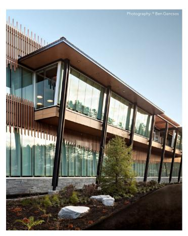
All systems can be flush glazed from either the inside or outside. The weatherseal option provides an alternative to SSG vertical mullions for Trifab® VersaGlaze® 450/451/451T. This ABS/ASA rigid polymer extrusion allows complete inside glazing and creates a flush glass appearance on the building exterior without the added labor of scaffolding or swing stages. Additionally, high-performance flashing options are engineered to eliminate perimeter sill fasteners and associated blind seals.
