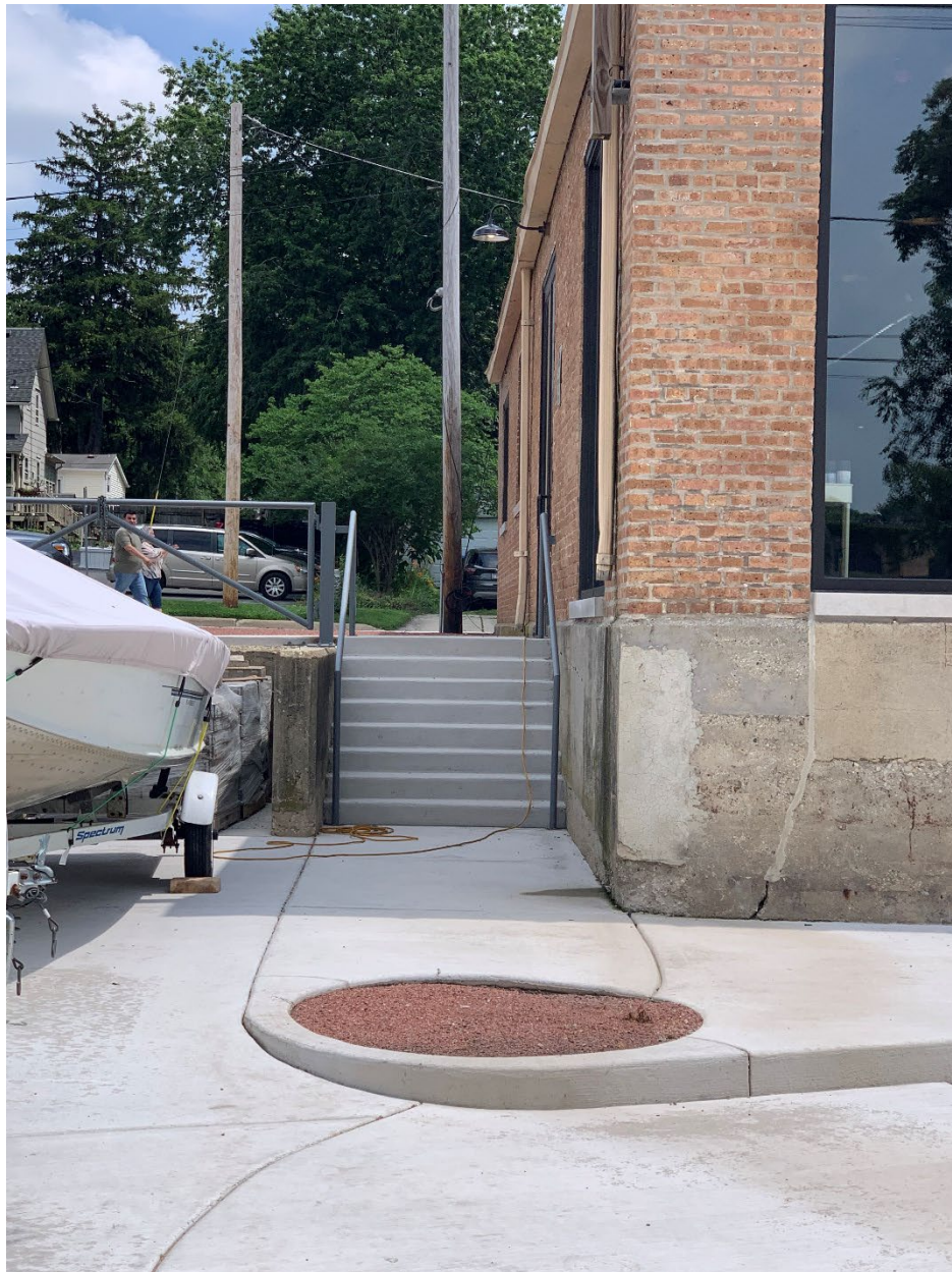
Railing that is currently installed
