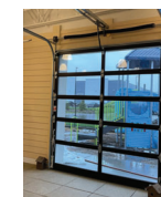
OVERHEAD DOOR MANUF : MIDLAND GARAGE DOOR MODEL : FULL VIEW FRAME : RIBL ALUMINUM COLOR : DEEP BRONZE GLASS : 1/2" INSULATED - TEMPERED LOW E-COATING
