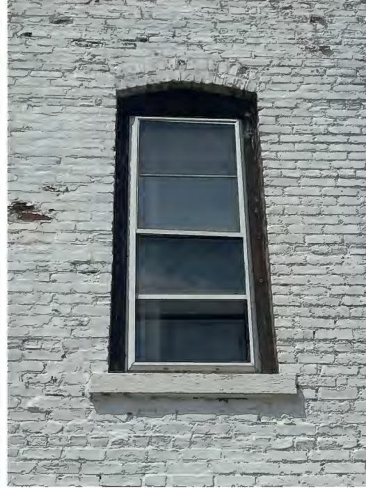
Side /South Facing
