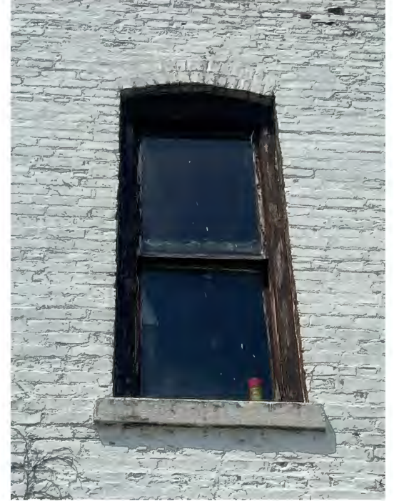
Side /South Facing
