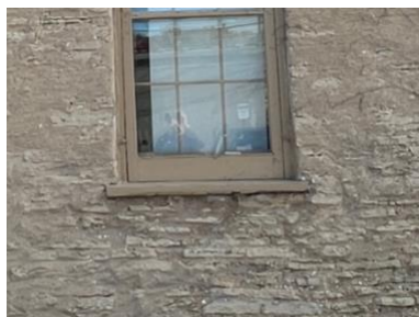
Figure 18. Open voids in the windowsill masonry.
