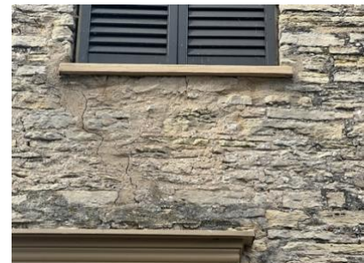
Figure 1. Cracking mortar above the front door on the East elevation.
