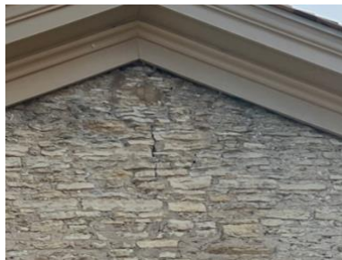
Figure 17. Close-up highlights cracked mortar joints.
