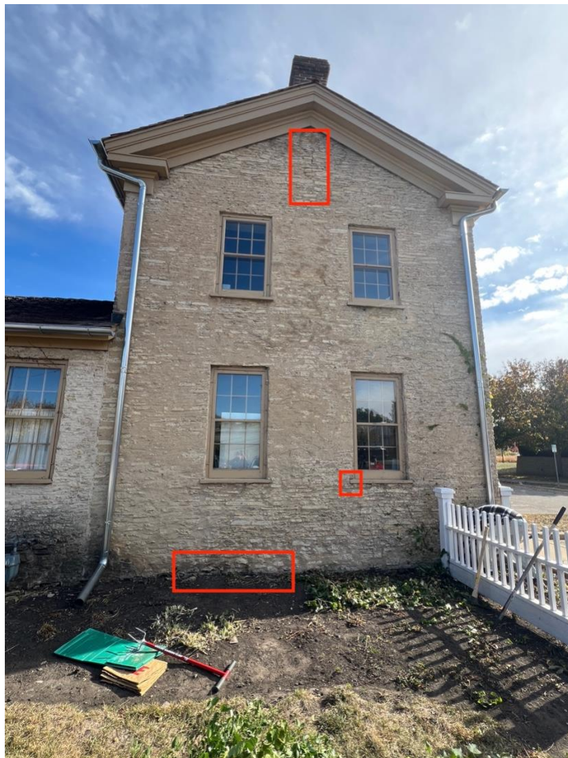
Figure 16. Main house's West elevation with visible issues in windowsills and foundation.
