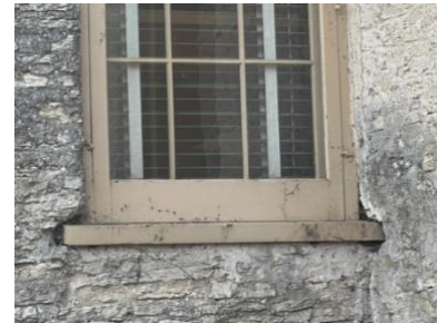
Figure 13. Cracking mortar detected, requiring injection to fill voids – 1 floor
