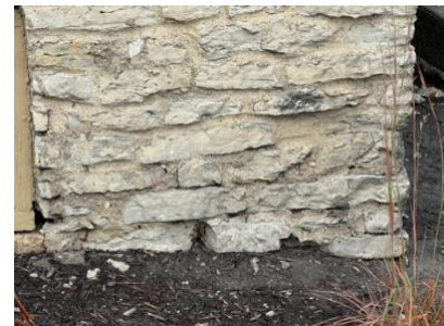
Figure 3. Visible foundation instability in the East elevation's base structure.
