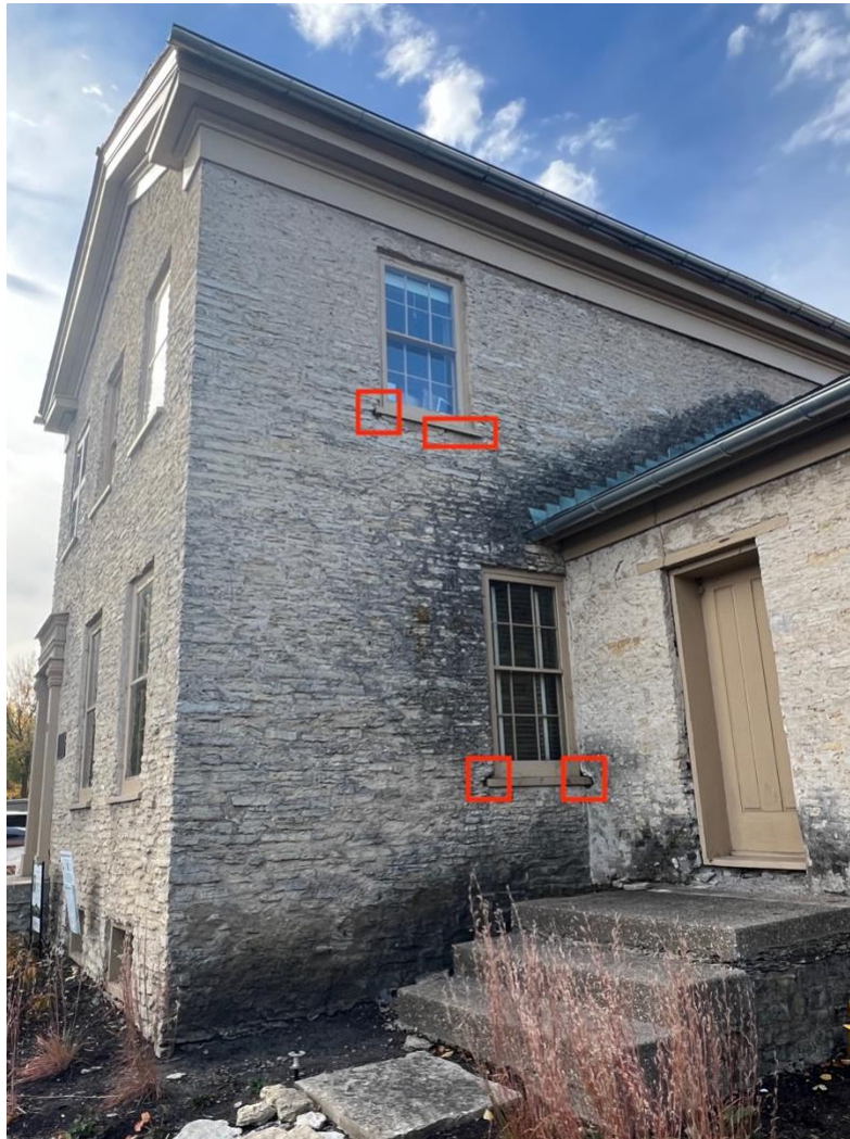
Figure 12. North elevation showing areas with open voids.
