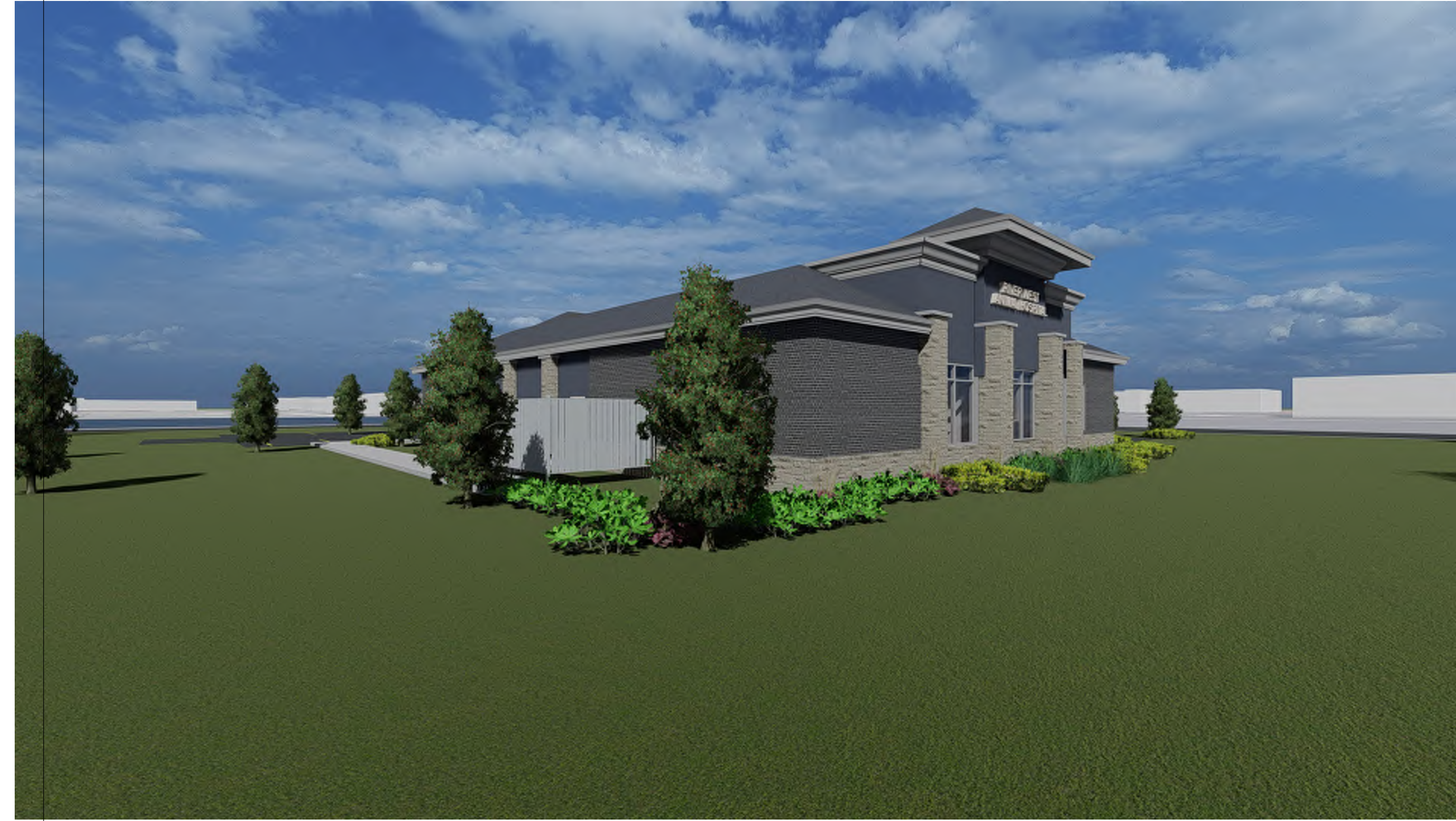
VIEW FROM ROUTE 64 WESTBOUND
