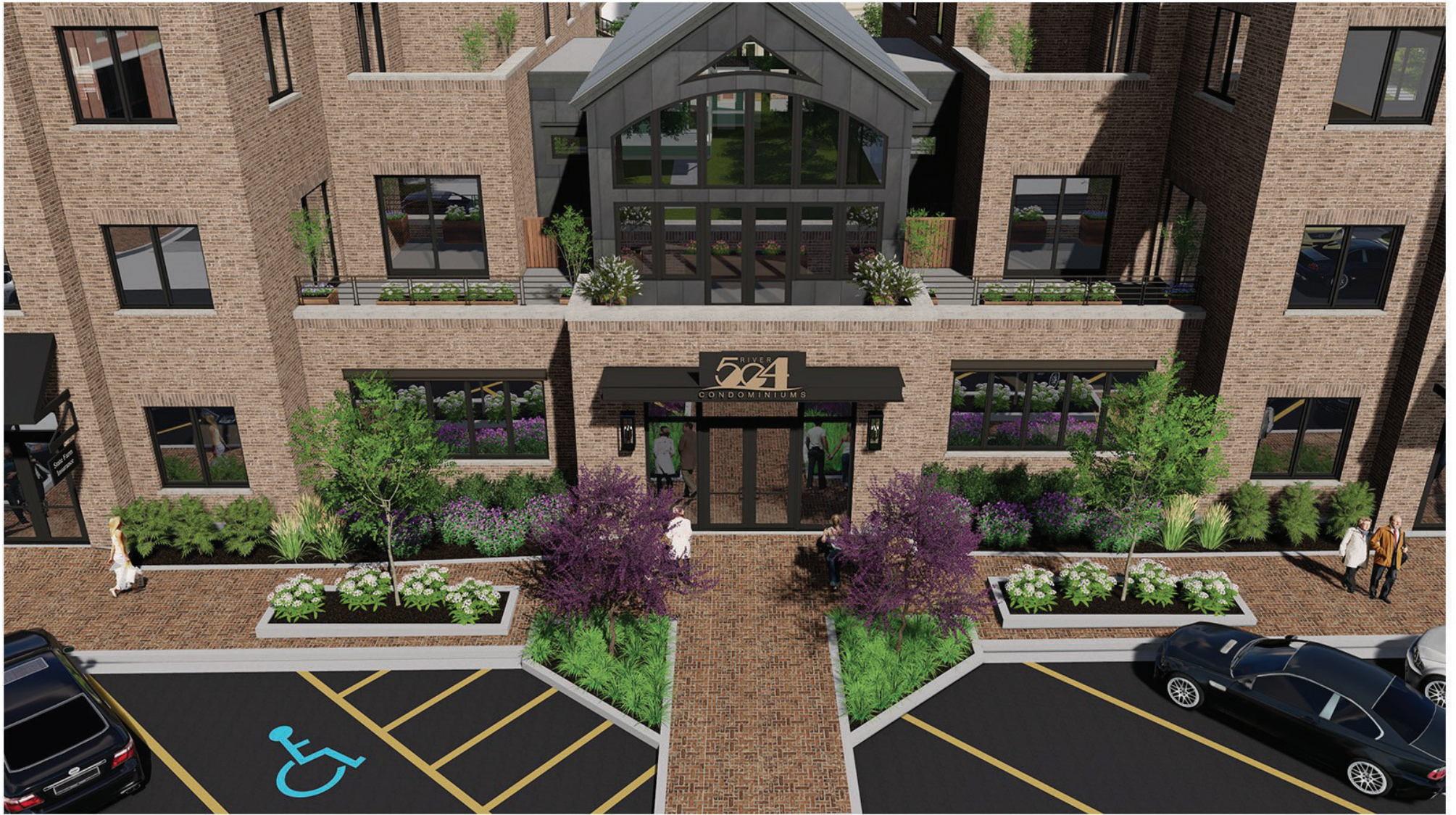
River 504 - West Elevation Center Entry
