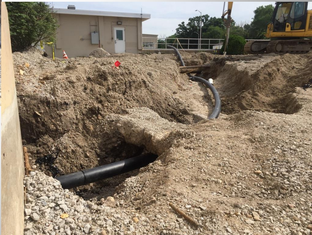
HDPE Digester Gas Line
