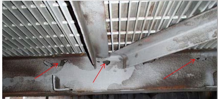
Prior To Repairs
