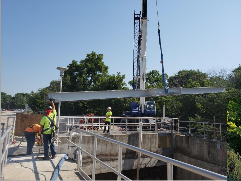
Lowering Mixer Bridges into place
