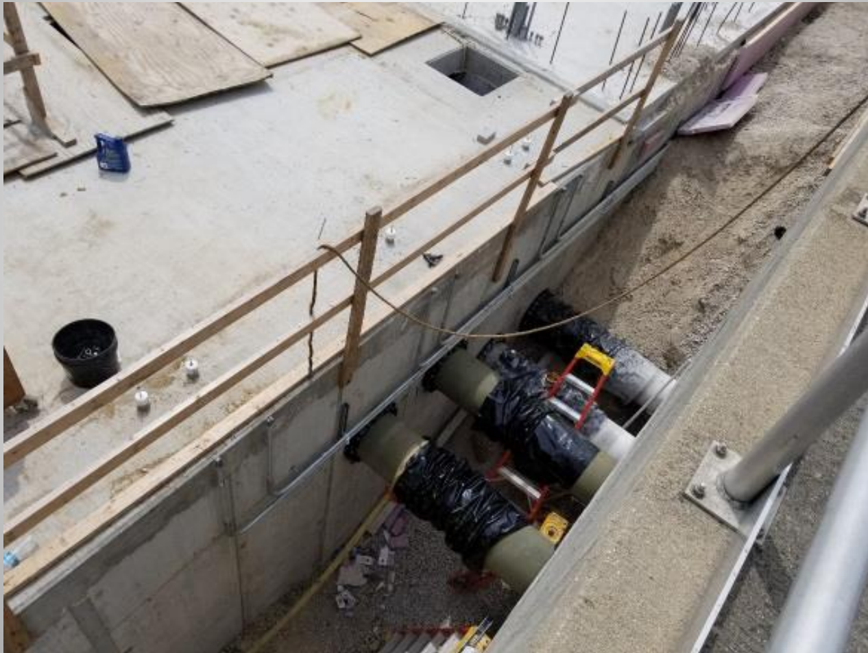
16" Pipe connection Between Pump Station and Aeration Tanks
