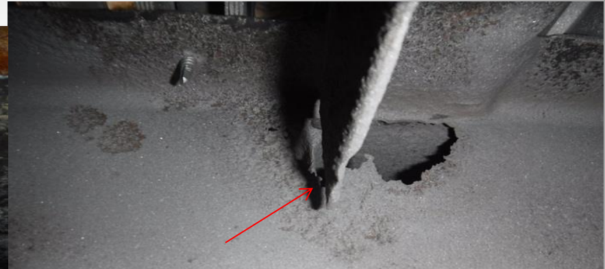
I-Beam holes in effluent box
