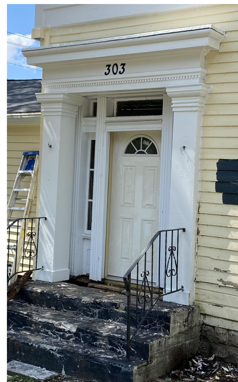
EXISTING FRONT ENTRY
