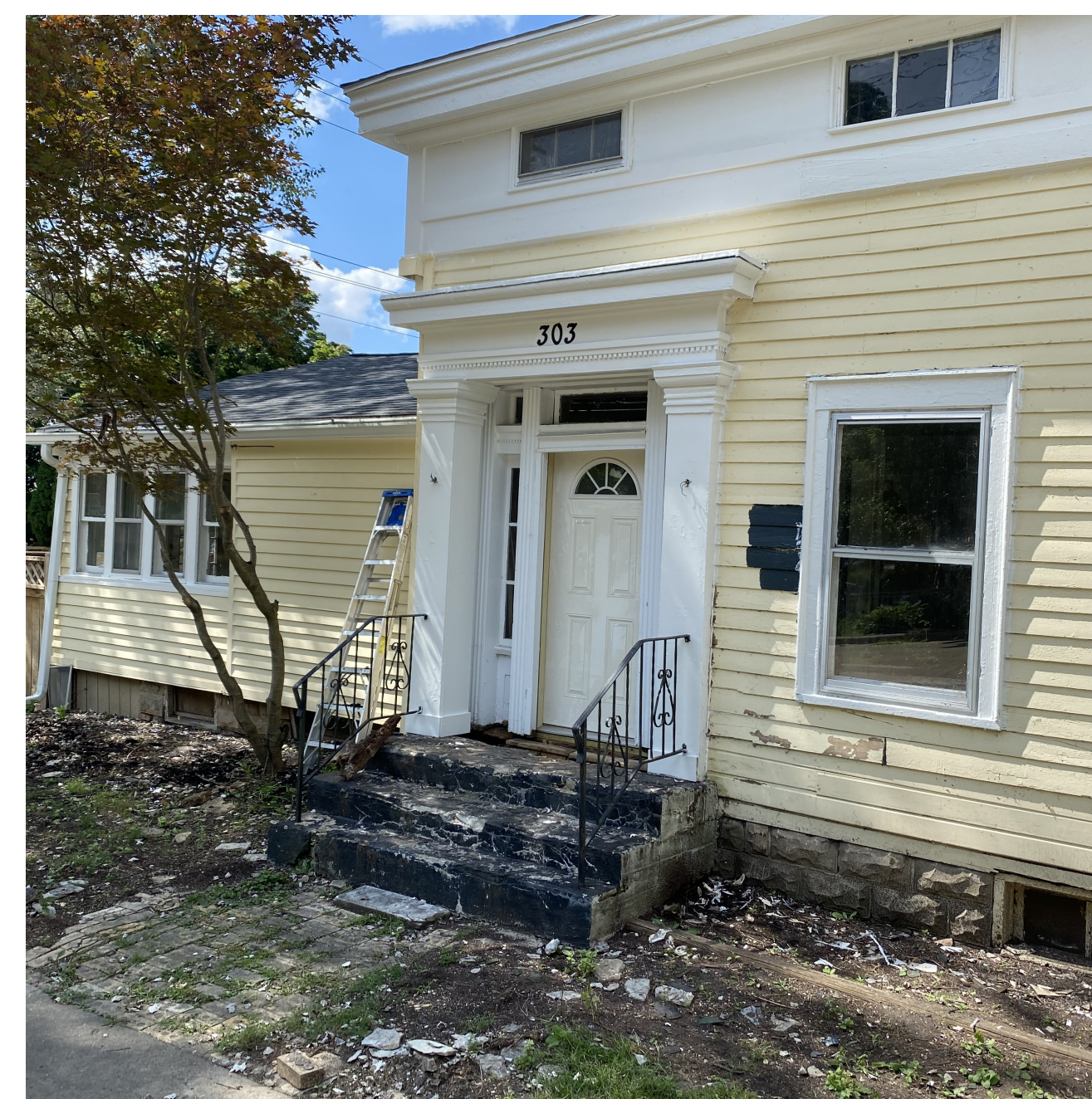
EXISTING ENTRY AND CORNICE DETAIL
