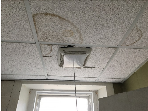
Roof leaks
