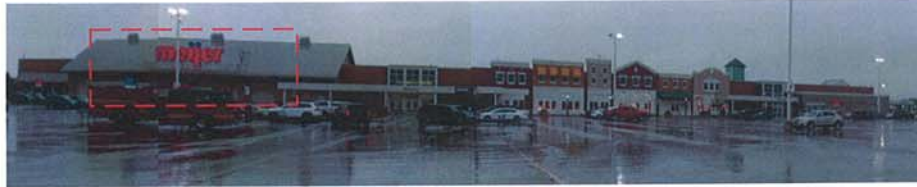
Existing Full Facade of Storefront
