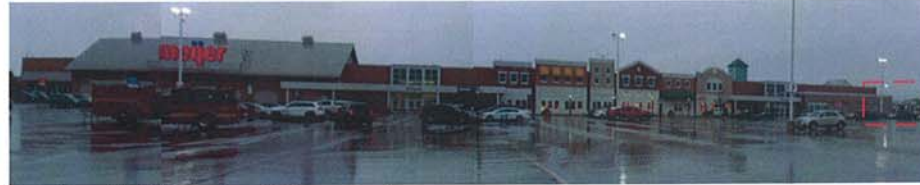
Existing Full Facade of Storefront
