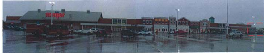
Existing Full Facade of Storefront
