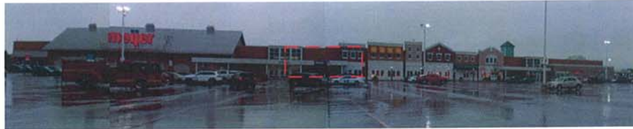
Existing Full Facade of Storefront
