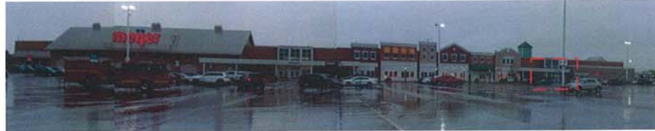
Existing Full Facade of Storefront
