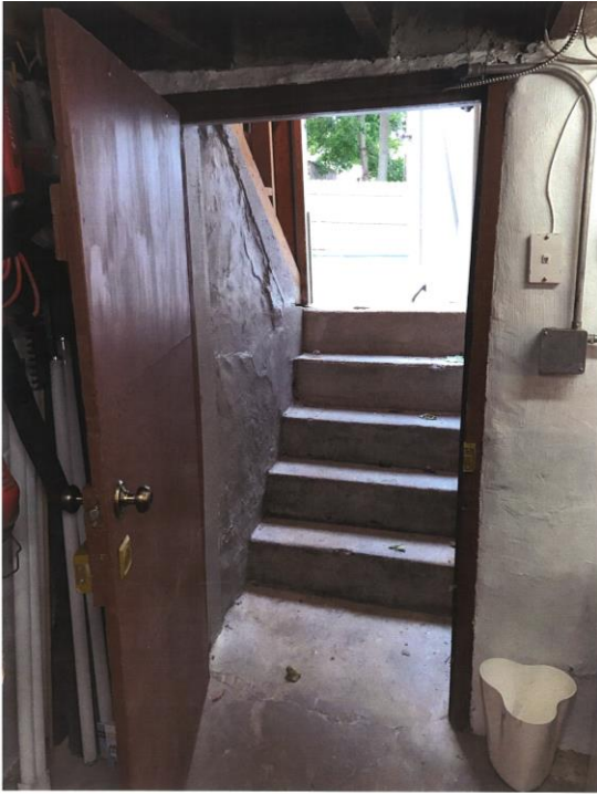
Entry from Exterior to Basement for Upstairs Apartment
