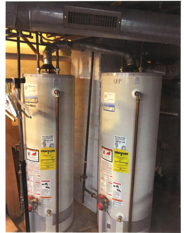
Separate Hot Water Heaters for Each Unit
