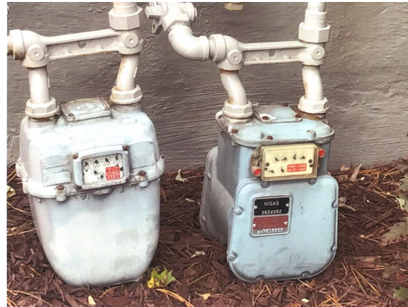
Separate Gas Meters for Each Unit
