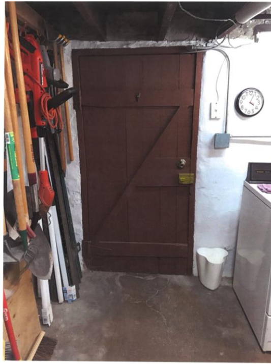
Entrance Door to Basement from Outside for Upstairs Apartment
