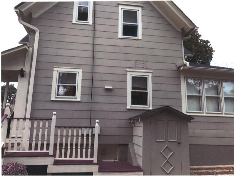
Showing Rear Access Entrance to Basement
