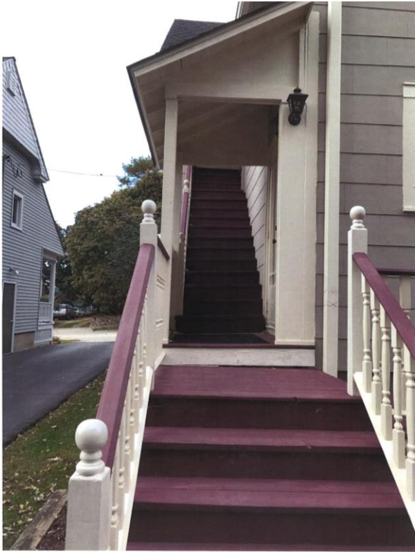
Separate Entrances in Rear of Building for Lower Unit and Upstairs Apartment
