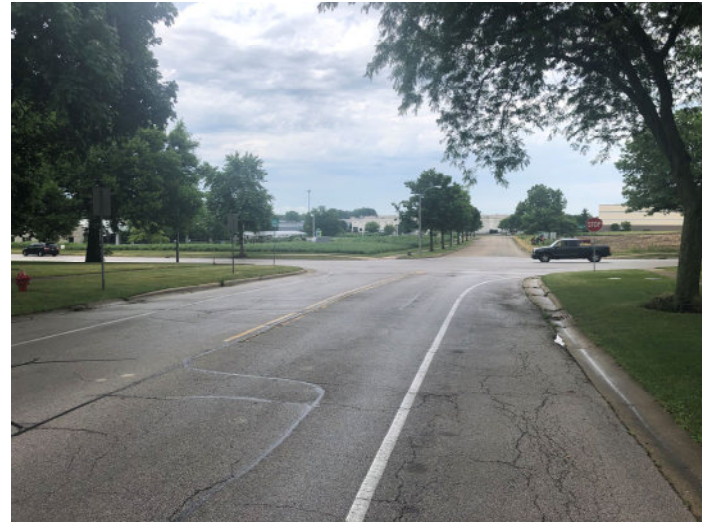
Looking east along Madison Ave at Tyler Rd
