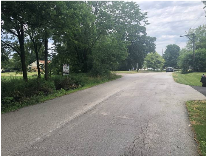
Looking north along Munhall Ave at Site Access
