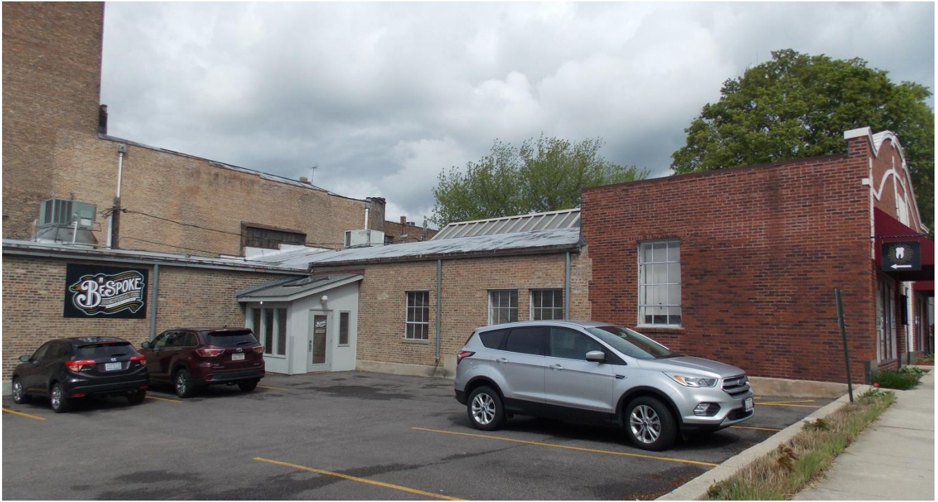
Portion of south side
