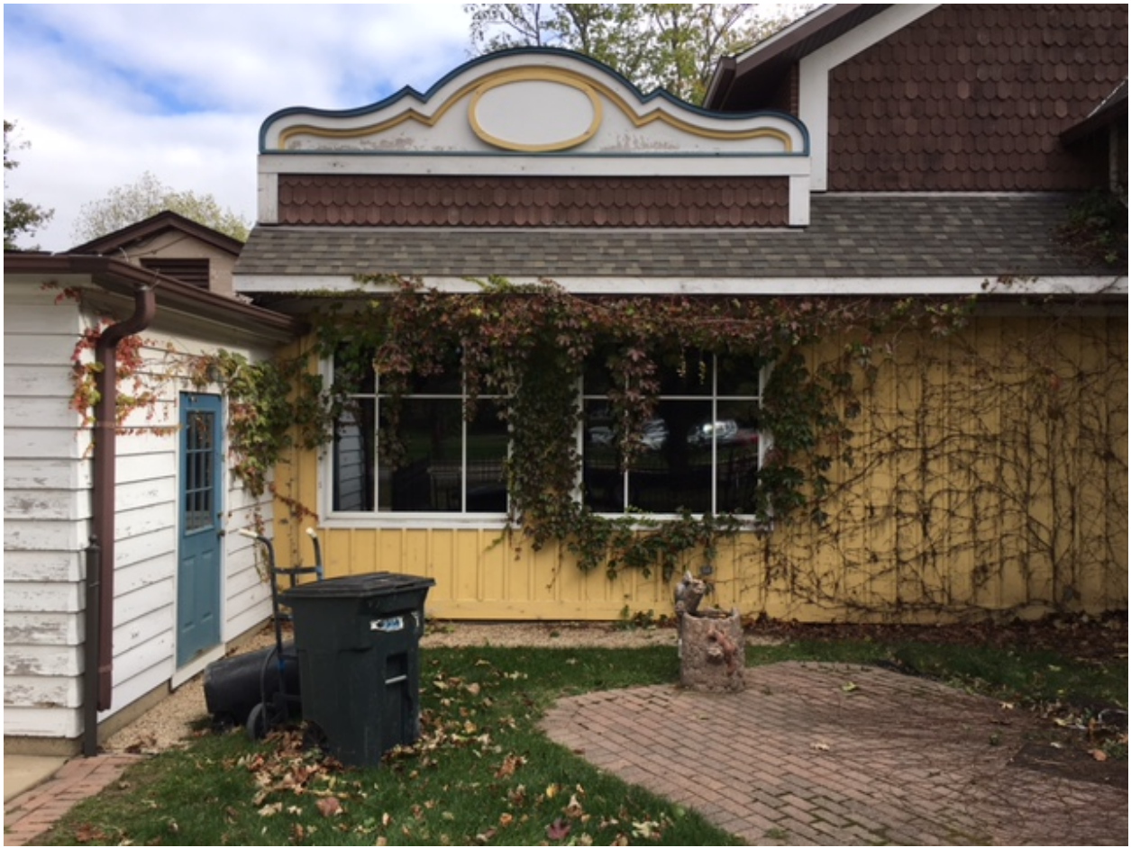
Existing west wall
