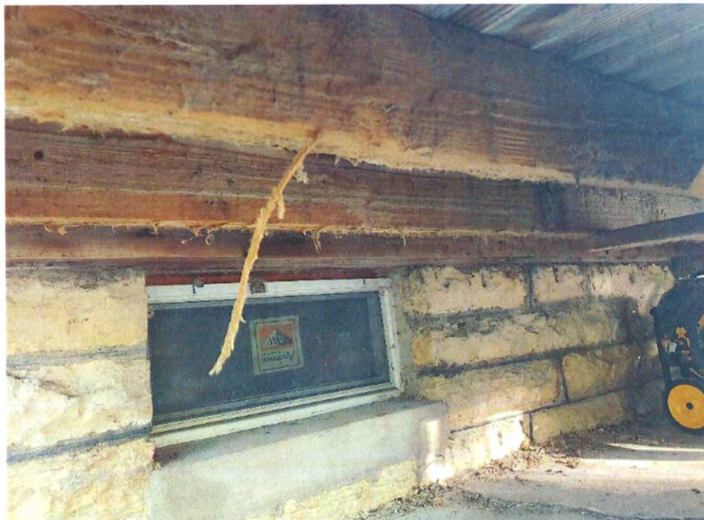
Wet, soft support beams supporting the deck:
