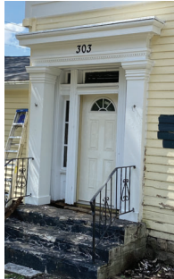
EXISTING FRONT ENTRY
