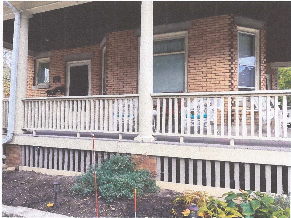
new rear railings designed to be similar to front porch using Lumberock products
