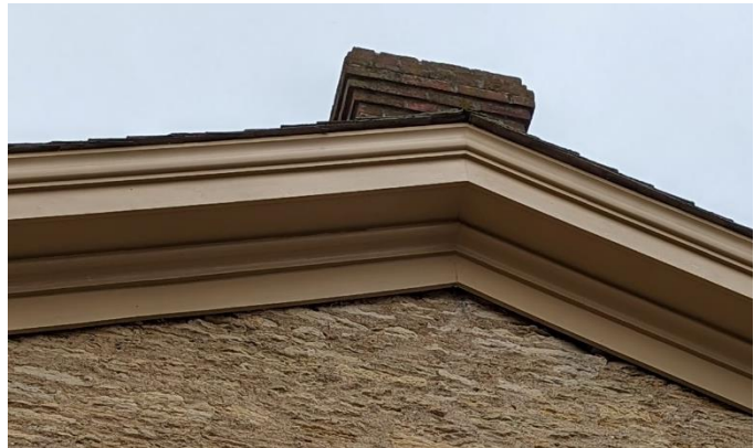
Replacement trim after completion.
