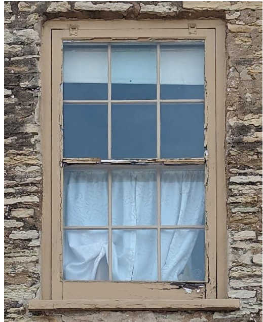
East elevation, second floor storm window.
