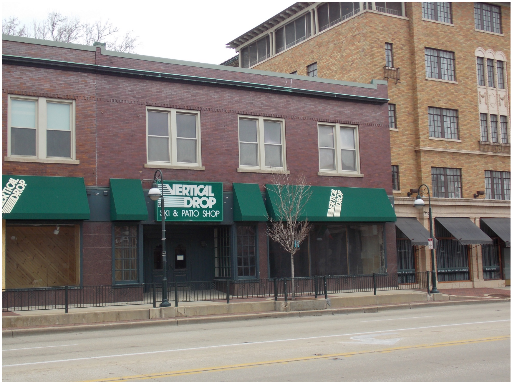
Existing east storefront proposed for renovation
