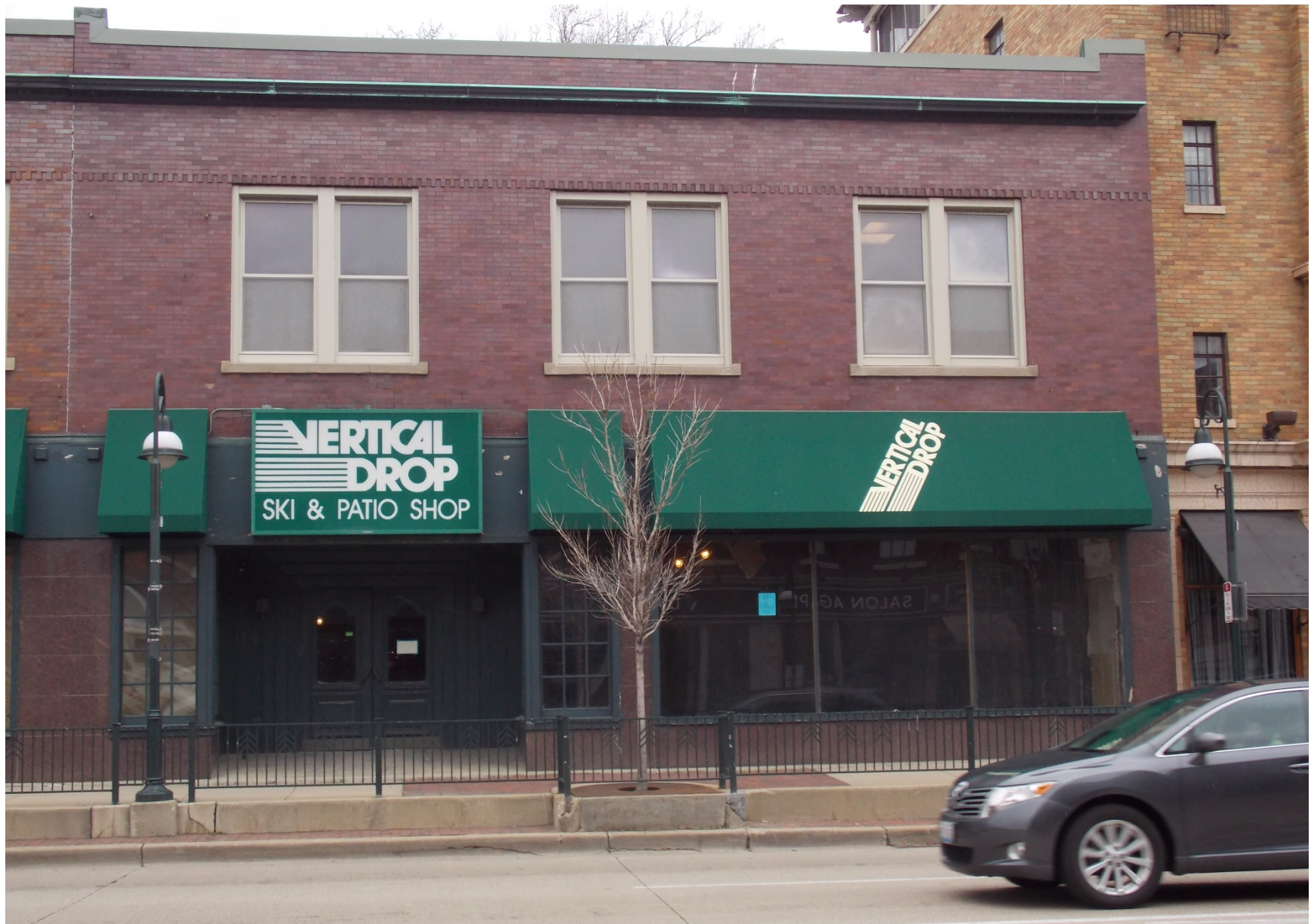
Existing east storefront proposed for renovation
