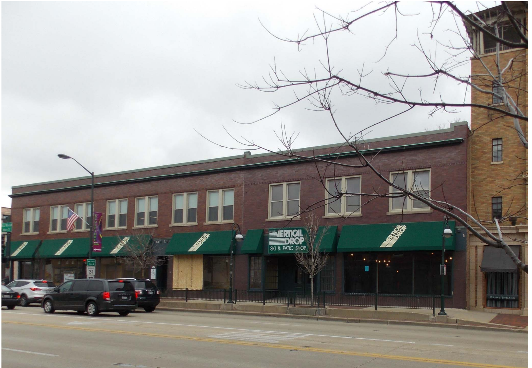
Existing former Vertical Drop storefront
