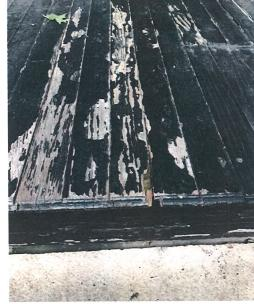
Porch areas require wood repair from excessive wear on steps.
