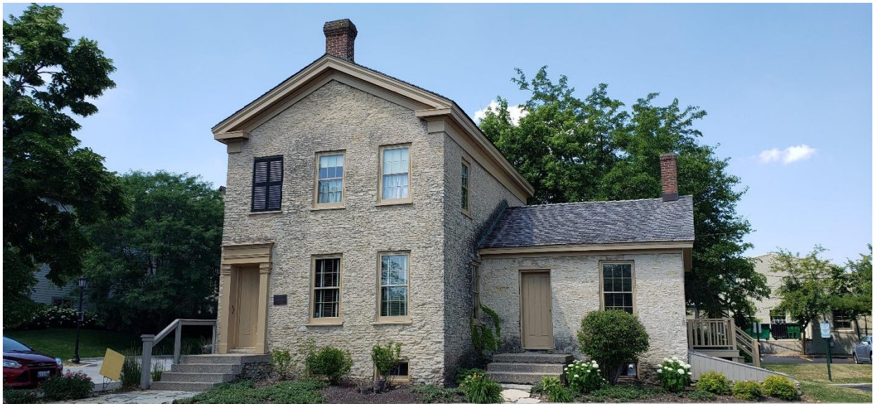
1850 William Beith House, East Façade
