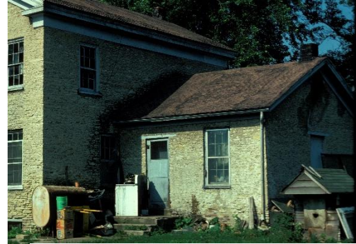
Some galvanized steel gutters c. 1970
