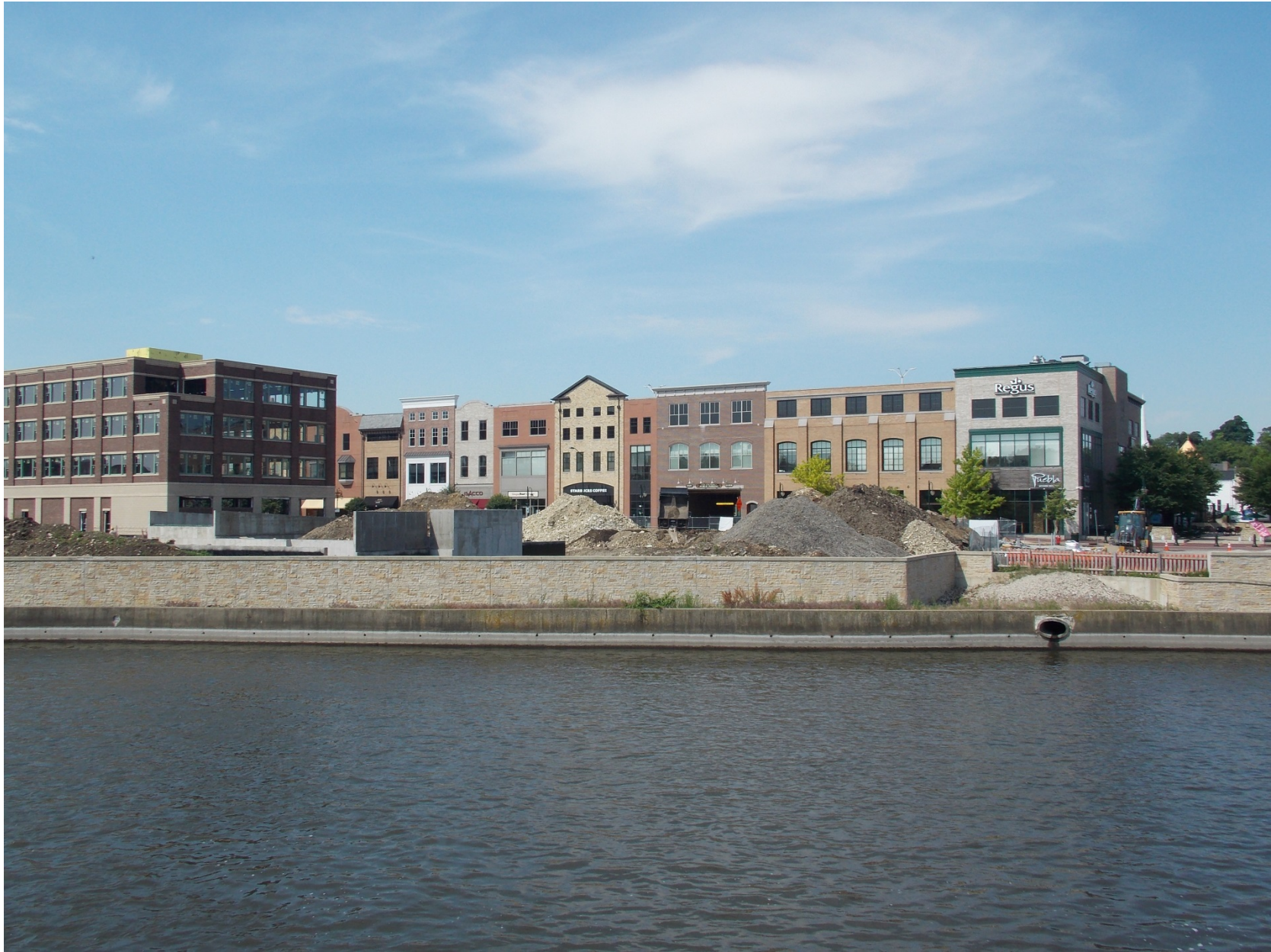
Building #2 site- June 2016
