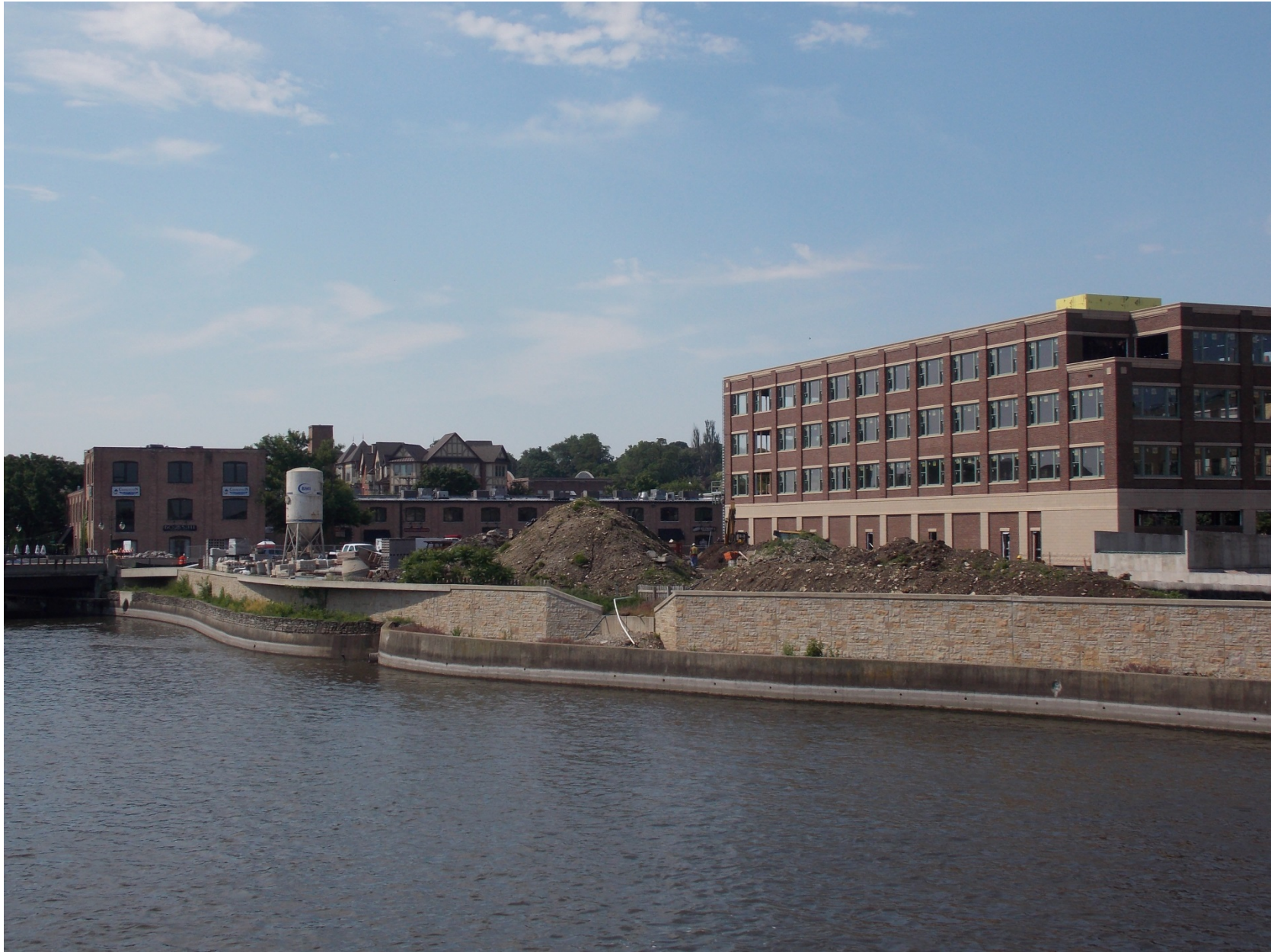
Building #3 site- June 2016
