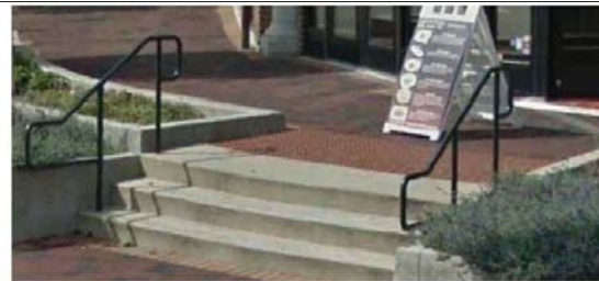
STEEL PIPE HANDRAIL FOR STAIRS
