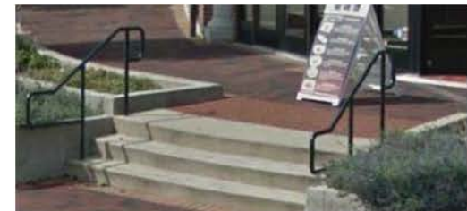
STEEL PIPE HANDRAIL FOR STAIRS
