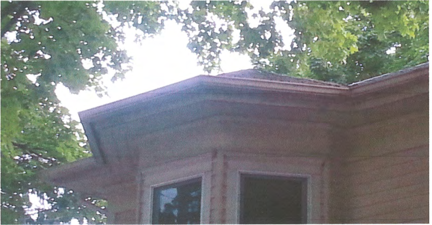
East Bay Soffit Detail
