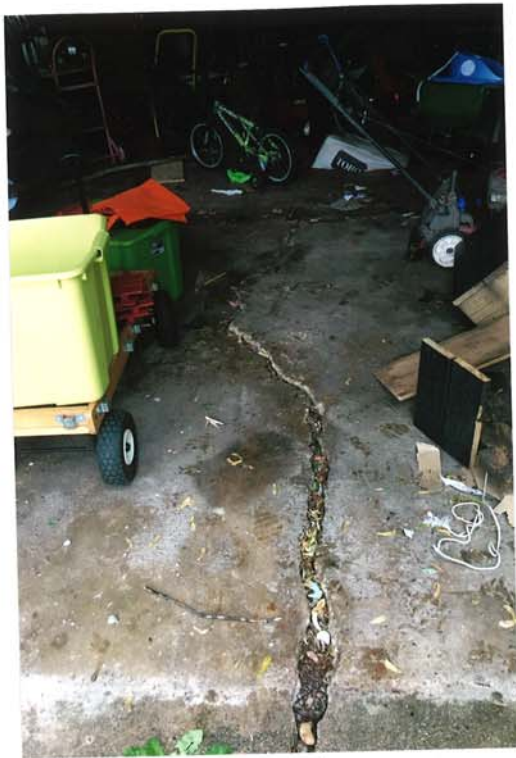
Foundation cracks ↑
