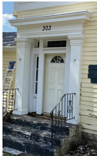
EXISTING FRONT ENTRY
