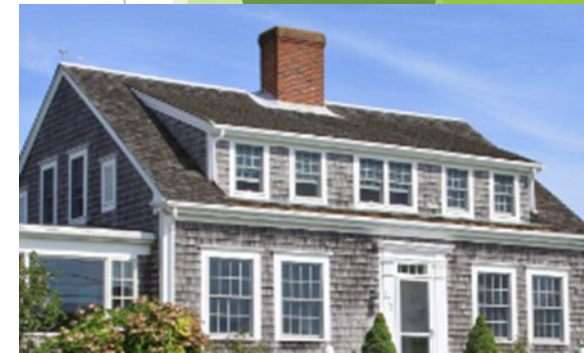
Typical Rear Yard View
