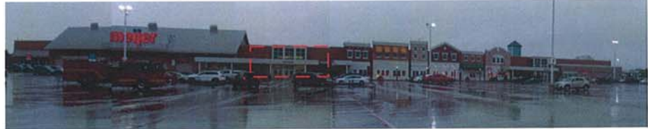
Existing Full Facade of Storefront
