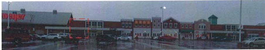
Existing Full Facade of Storefront
