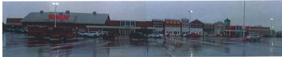
Existing Full Facade of Storefront
