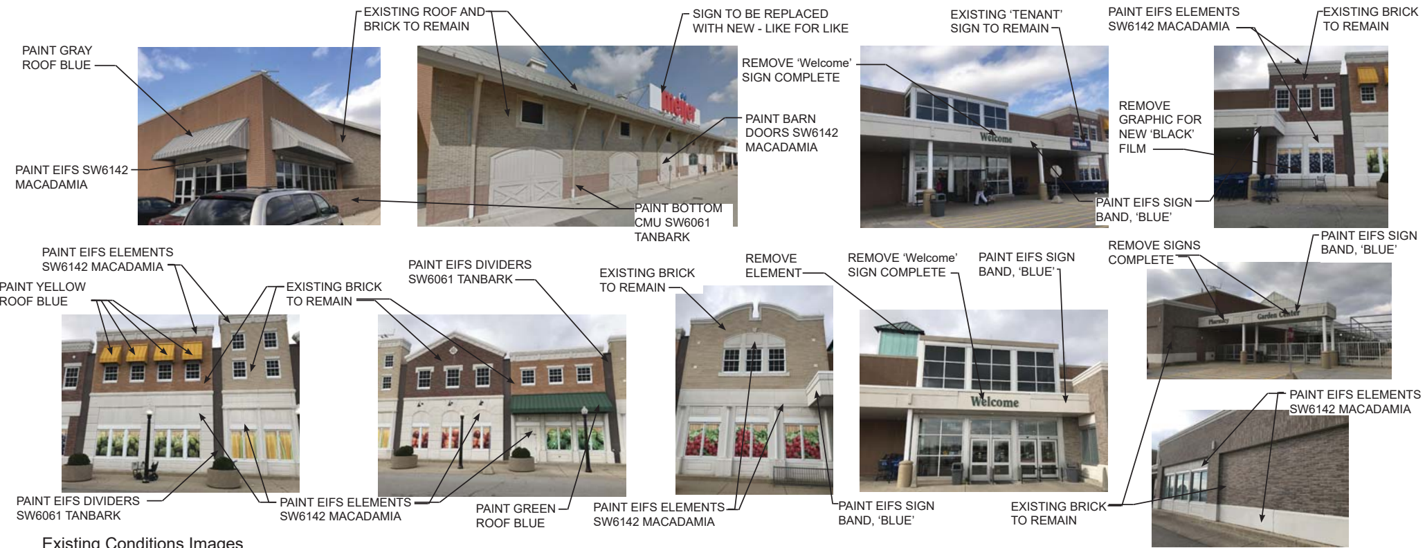
Existing Conditions Images
