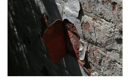
The face of the brick is failing in places and the paint is peeling because of it. It needs the attention of a masonry expert to preserve the brick and provide a decent surface to paint. These are just a couple small spots. There is a larger spot that was too high to be easily photographed.
