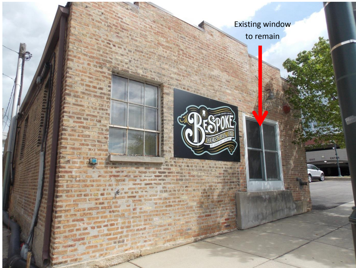
Portion of south side (Walnut Ave.)
