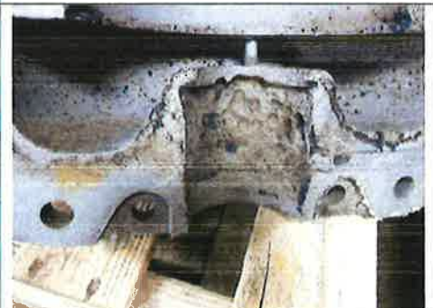
Heavy pitting in shaft bearing journal
