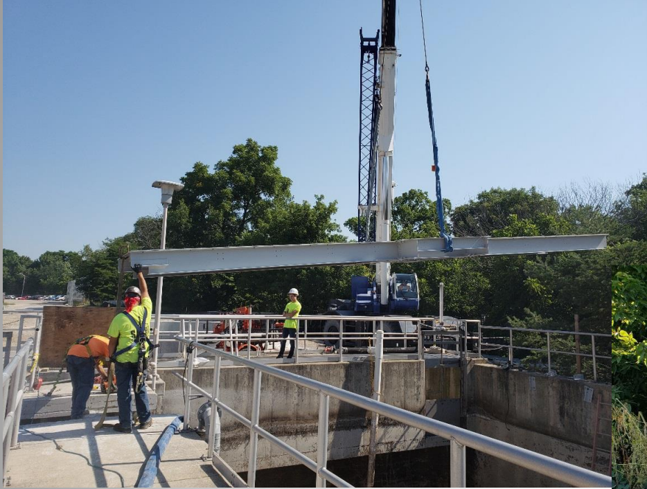
Lowering Mixer Bridges into place
