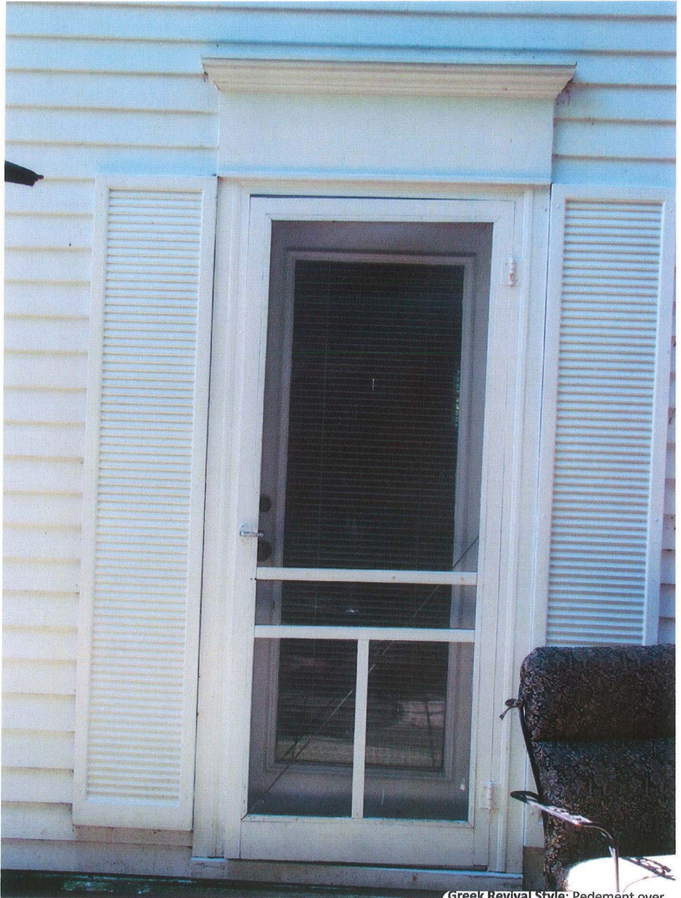
Greek Revival Style: Pediment over window and doors
