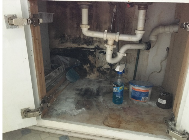
Mold and rot under kitchen sink
