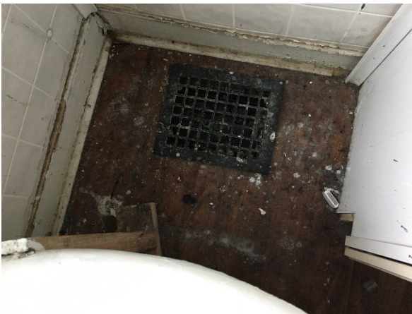
Mold in bathroom, likely inside duct work also
