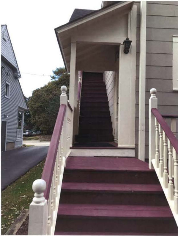
Separate Entrances in Rear of Building for Lower Unit and Upstairs Apartment
