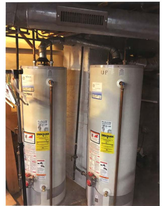
Separate Hot Water Heaters for Each Unit
