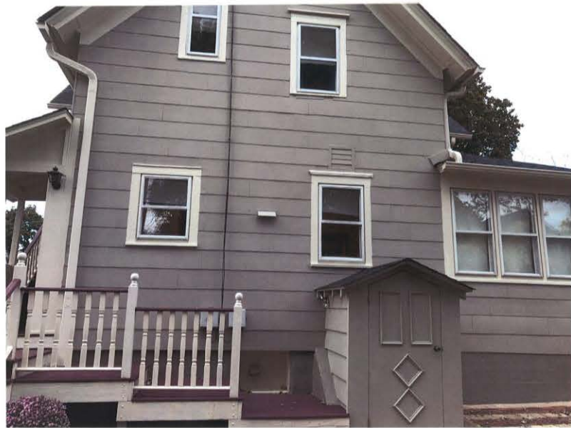
Showing Rear Access Entrance to Basement
