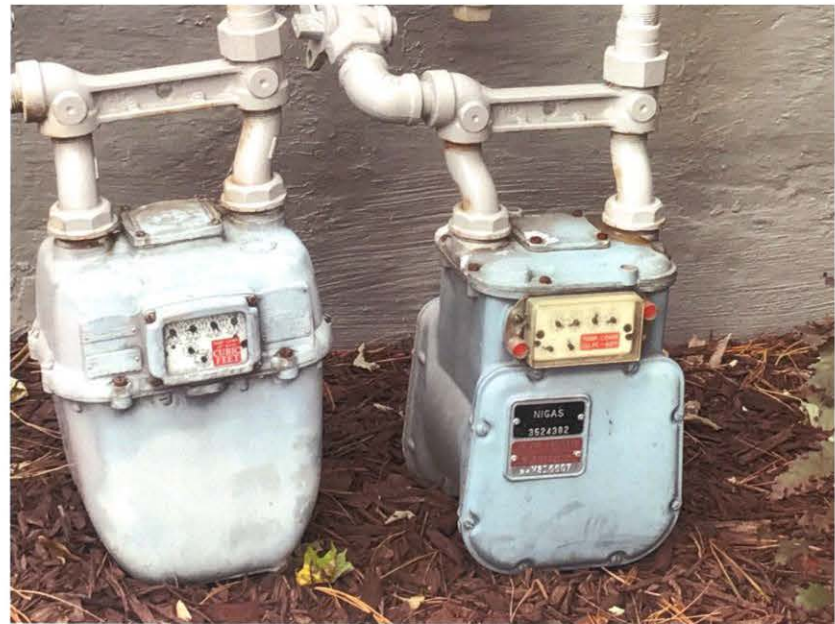
Separate Gas Meters for Each Unit
