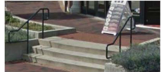
STEEL PIPE HANDRAIL FOR STAIRS
