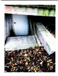
Plandscape also created a retaining wall on the backside of our Community Resource Center. For years, whenever there was a soaking rain, water would flow down the stairs that led to the basement of this building and end up creating large puddles on the basement floor. This moisture often wreaked havoc with our computer systems and hindered us from using the floor space as storage. With the new retaining wall we have a much drier space we can utilize.
